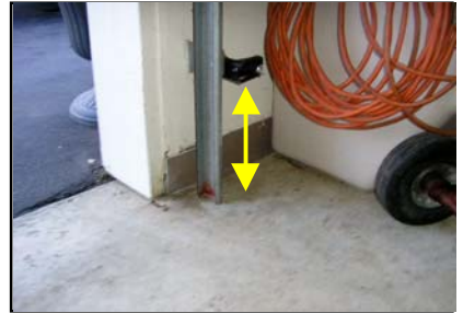
6 " max recommended for door sensors.
