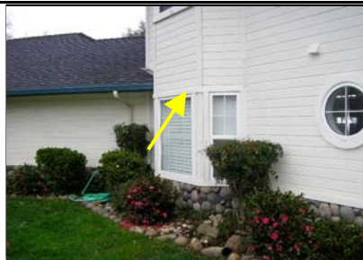
Caulking is recommended above window & siding trim.
