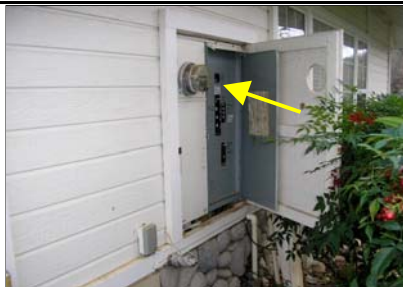
Main electrical disconnect.
