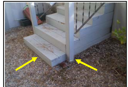
Earth to wood contact will accelerate wear to step & support post material.
