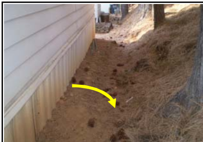
Positive grading & ditch noted along rear of house.
