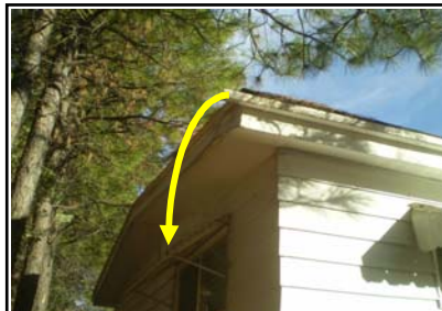
Open ended gutters are discharging roof run-off next to house.
