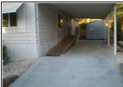
Attached carport/ parking
