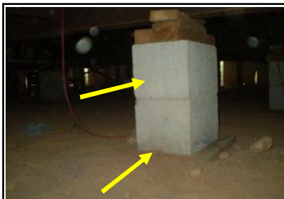
House support is concrete block on wood pads.
