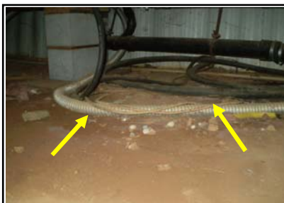
Electrical feeder cable & wiring noted laying on soil in crawl under house.
