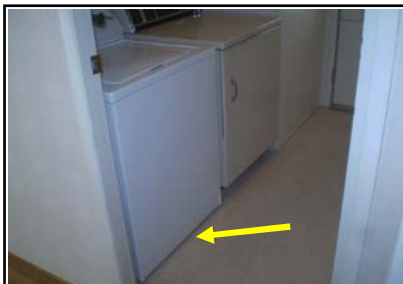
Drain pans are recommended under interior washers.
