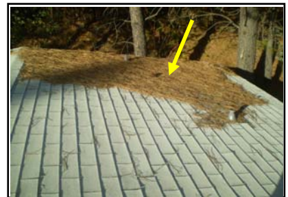
Recommend keeping debris cleared from roof surfaces.
